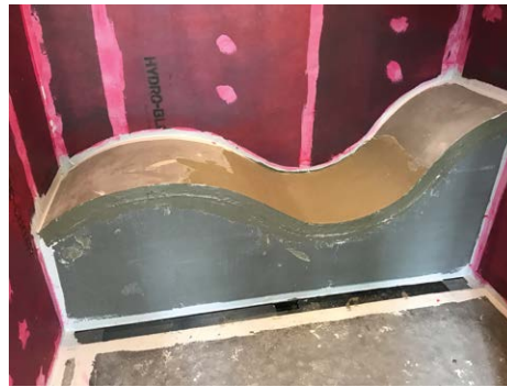
Custom curved residential shower bench created with HYDRO-BLOK 2" Building Board - see it built and installed on the HYDRO-BLOK YouTube Channel!
